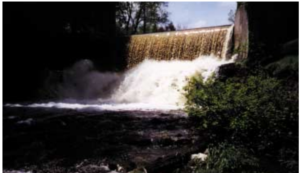
The Progreston Dam, 14 feet high, may have major thermal heating impacts on the lower river.
