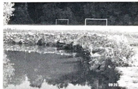
Finished! Stumps placed at the water line and the rock covered bank.
