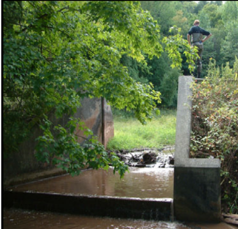
A 2.3 m dam removed over 3 years from Rogers Creek by CRAA, CVC and MNR.
