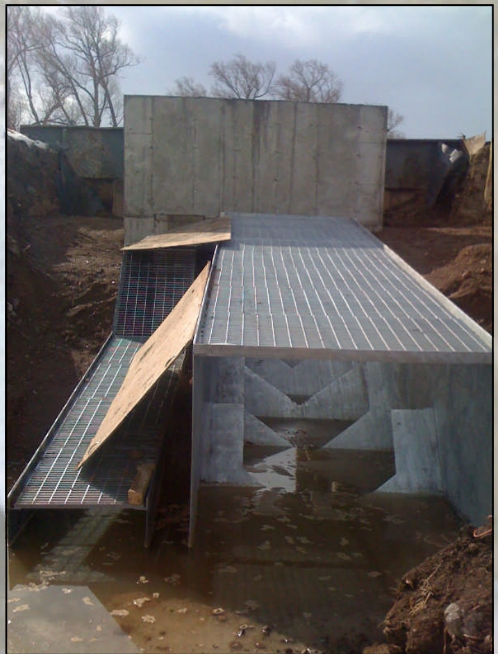
Looking into the new fishway from the entrance. The Denile fishway on the left is the old fishway with new baffles that pass 4 times more water. The ladder on the right is new and is six feet wide and almost 7 feet tall. Fish swim through the ladder into a collection cage for sorting.
