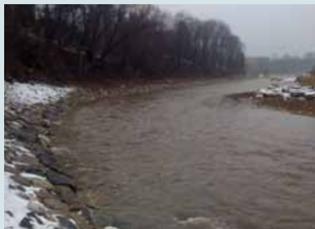
CRAA was involved in the public design phase of this huge bank stabilization project built by Mississauga over the winter of 2011 downstream of Britannia Road
