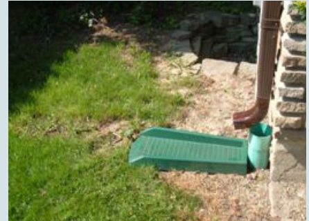
The disconnected downspout at the Kendell residence.
